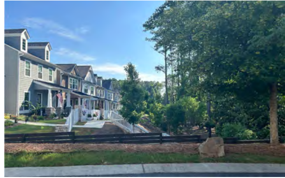
View from driveway looking north.
