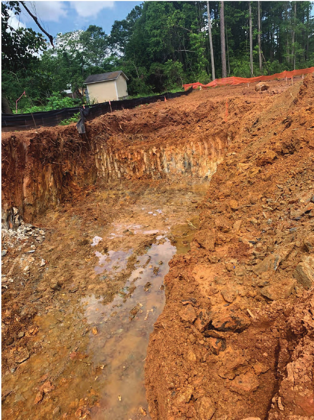
Ground Water Photos – Pond Wall B-1 July 8, 2020
