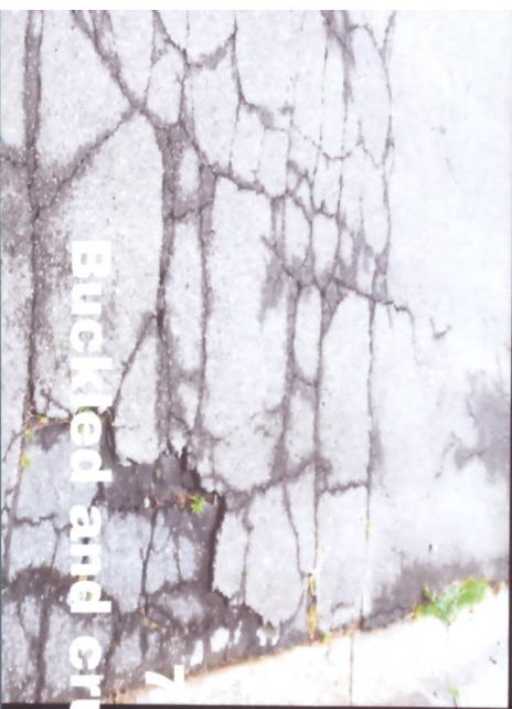
7 of 7 Buckled and crumbling pavement
