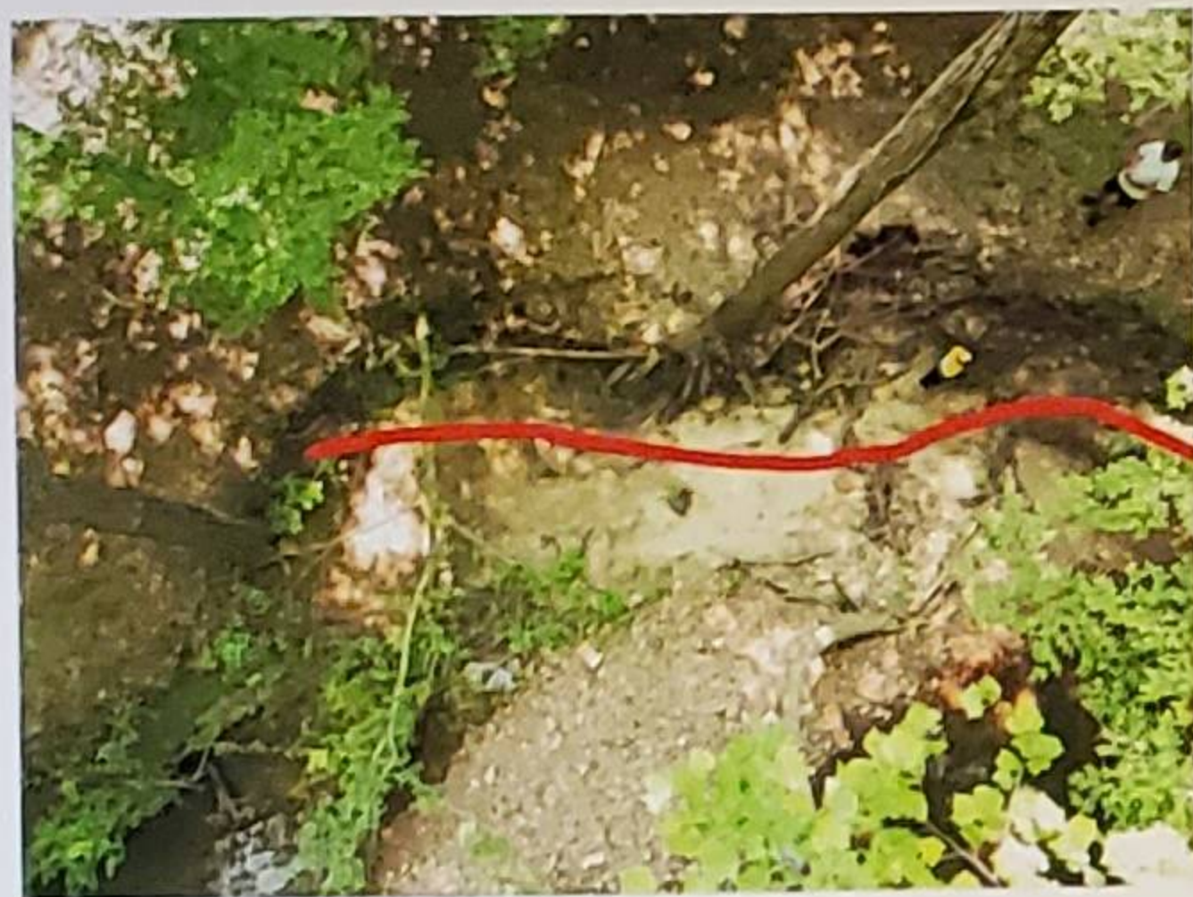
Change in edge of embankment
